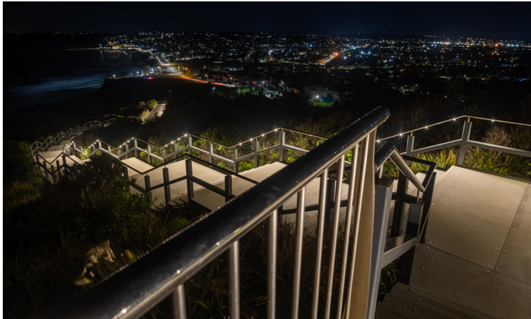
Walkway Honours Peter Treloar
